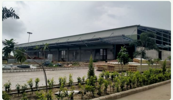
Telecom and Data Centers
